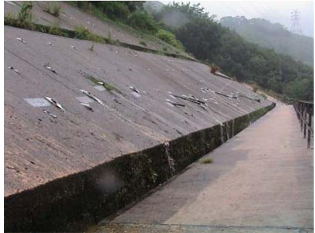
**Fig. 8.** A multiberm high slope with regular rows of raking and horizontal drains. Note the irregular flows pattern (Tsing Tsui Estate, HK).
