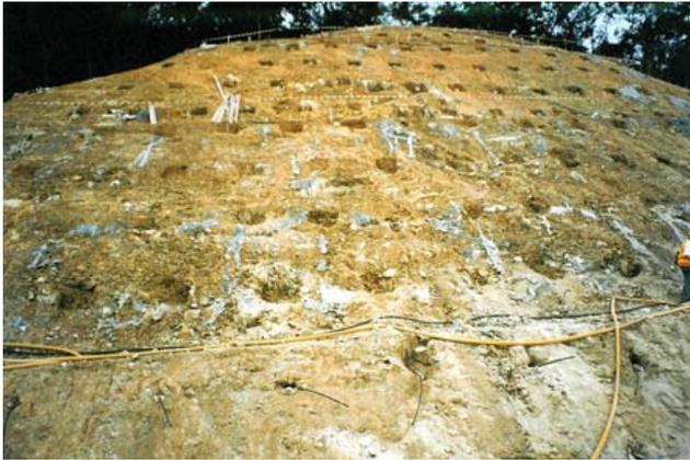
**Fig. 9.** Soil nails installed over a regular grid pattern of boreholes drilled throughout a volcanic saprolite profile.
