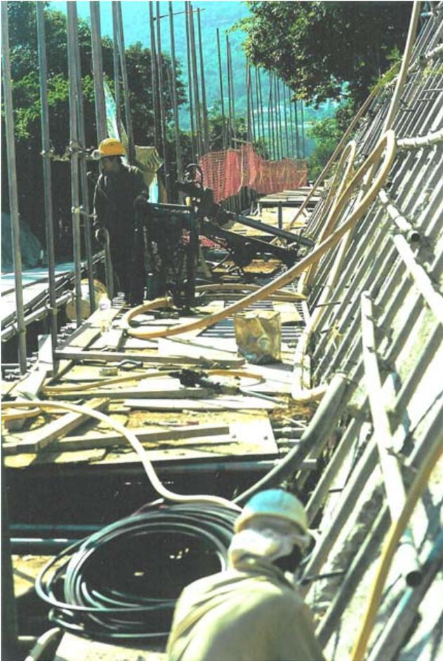
**Fig. 10.** A pneumatic rotary-percussive drill machine on a temporary platform set-up for the installation of soil nails and horizontal drains along a predefined series of rows.
